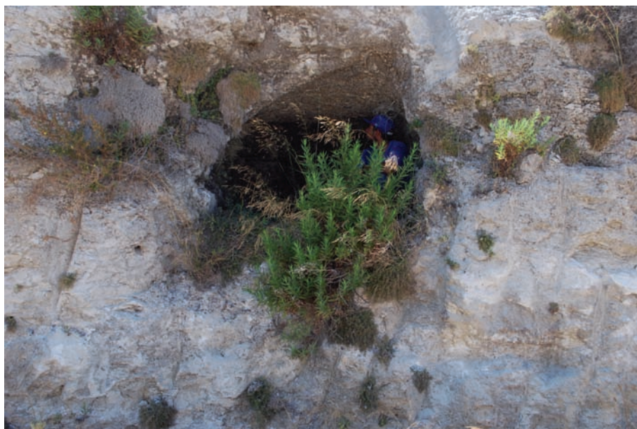
Fig. 8 CRS004, rock-cut chamber tomb destroyed by the construction of a modern street (©OREA & AUB, photo H. Genz)
